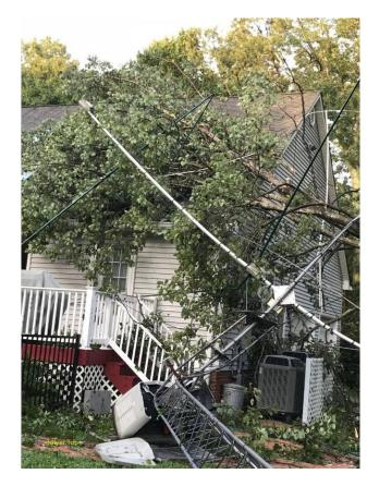
The "Tower Top" picture shows a tree on the house roof, wiped out generator, the tower top, the remains of a 4-element SteppIR, a 40m Moxon and the bent 2-inch dia., 1/4 inch wall, chromoly steel galvanized mast. The tree saved much more damage to the house by absorbing the falling top of the tower rather than the house.
