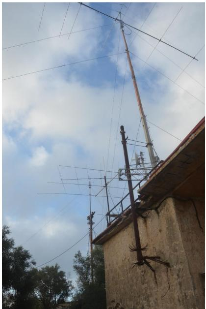
Multiple beams for HF at IB9T. There is also a 4-square for 40m, and other LF antennas.
