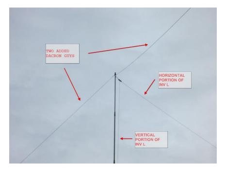
Figure 5. Top of Steppir showing inverted-L in place after being hoisted up.
