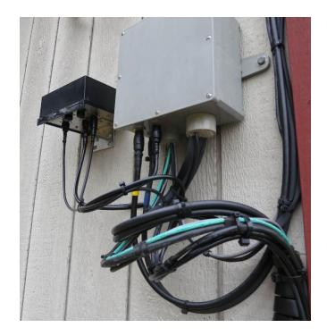
Above photo shows the RCS-4 relay box on the left of the conduit junction box mounted on a backyard shed. The RCS-4 relay box allows switching of one feedline between the BOGs and the K9AY loop. The loop-on-ground antenna is located in the front yard and uses a separate RG-6 feedline to the shack.
