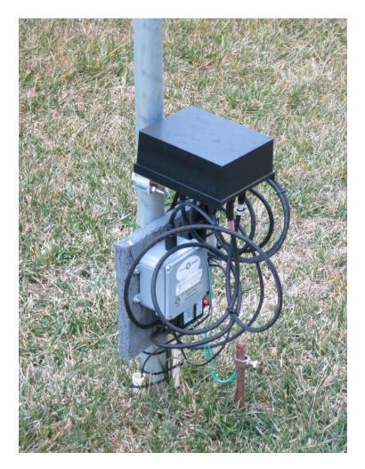
Beverage-on-ground hub, showing balun, feed and reflection transformers, and RCS-8V relay box.
