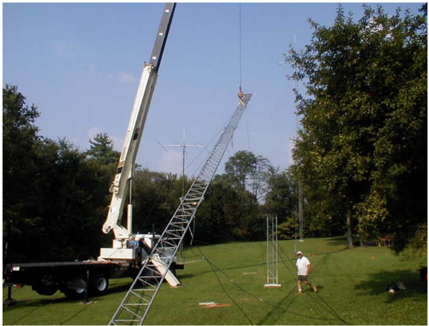
The first tower goes up, guy wires and all
