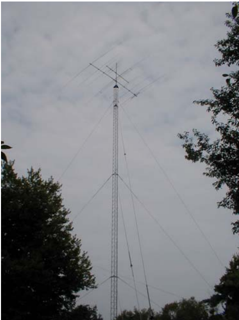
Tower #2, with the Skyhawk and 6M yagi
