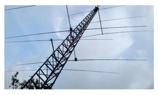
The 80 meter array (not a great picture) is made of two full size aluminum verticals and there were about 130 radials under the array. Tom NI1N loves radials:
