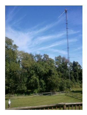
With Mike standing at the 134 foot level on the top of the tower, we rigged my stainless steel cable tram line, tensioned it to about 800 pounds. Mike attached the EF-180C to the tram pulley and we lowered it to the ground. While Mike waited on the tower, I replaced both element tips, riveted them in place, and hauled the antenna back to Mike using my lawn tractor to pull it back up the tram line. Mike reinstalled it on the mast, raised the mast, secured it all and I was back on 80m big time!
