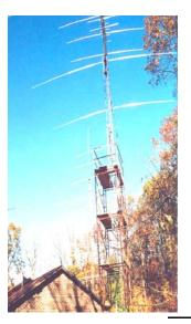
Photo at left shows W8ZA's crank-up with scaffolding in place below the 3-element 40-meter Yagi.
