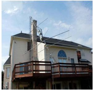
This picture shows what greeted us on our return from a trip to Russia on August 26 - apparently two days after high winds had hit parts of Clarksburg MD. The tower was 50 feet of Rohn 25G, of which the lower 30 feet were securely bracketed to the masonry chimney. It buckled just above the topmost bracket.
