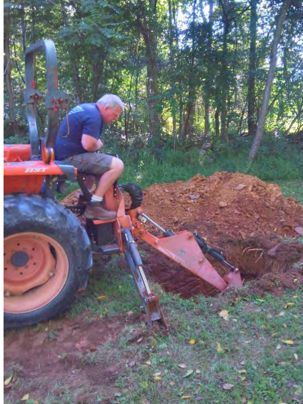
Matt Hackett from Mobile Equipment Services mans the backhoe.
